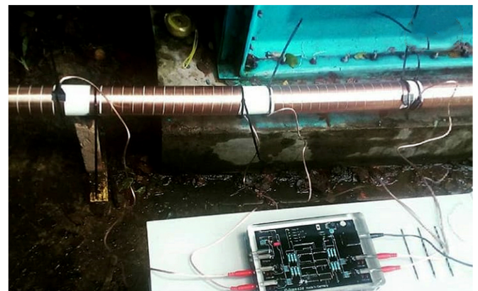
Picture 4. Vulcan installation process at the main incoming water line.
